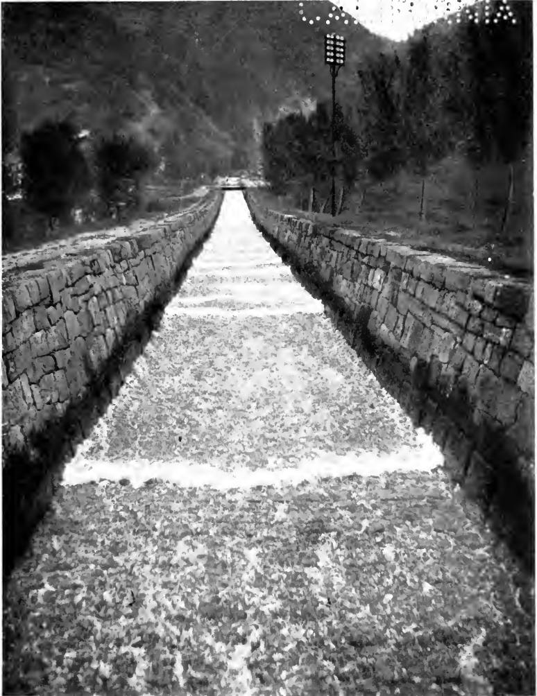
ROLL-WAVES IN THE GRÜNNBACH CONDUIT, LOOKING UP-STREAM.
